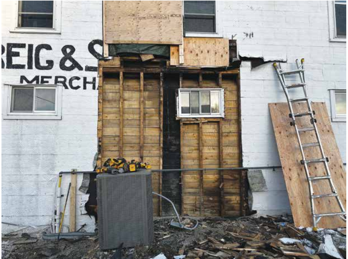
▲ The fire started between these studs, reached up to the second floor and then spread. PHOTO BY TONY AGUILAR.
